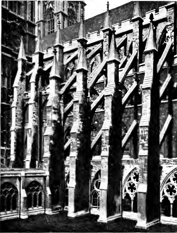
34. Buttresses to Nave, Westminster Abbey.
